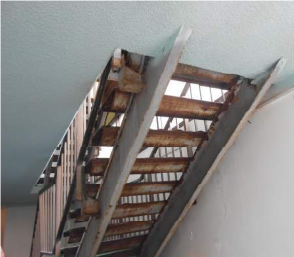
Photo 11: DSCN0481– Typical steel stair rusting
