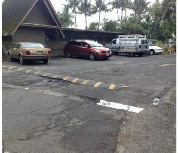
Photo 2: IMG_2445 – Deteriorated pavement at entry parcel
