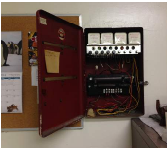
Photo 23: IMG_2450- Fire alarm control box
