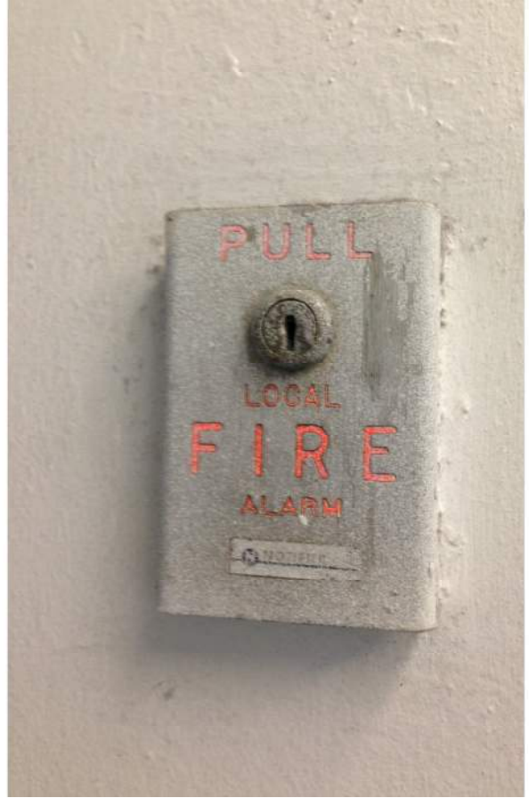
Photo 22: IMG_2463 – Fire alarm pull box
