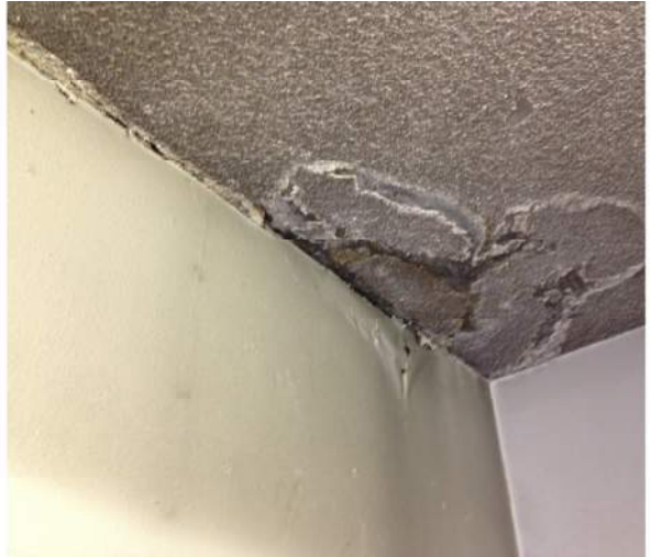
Photo 8: IMG_2519 – Water Damage, cracking and efflorescence at ceiling
