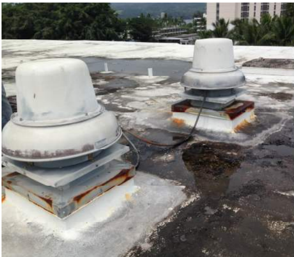
Photo 19: IMG_2569 – Exhaust Fans
