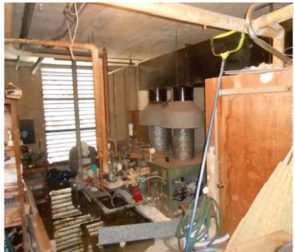
Photo 20: DSCN0461 – Heater/Boiler Room
