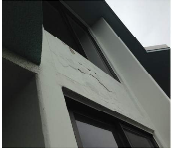
Photo 6: IMG_2523– Spalling at Exterior Wall
