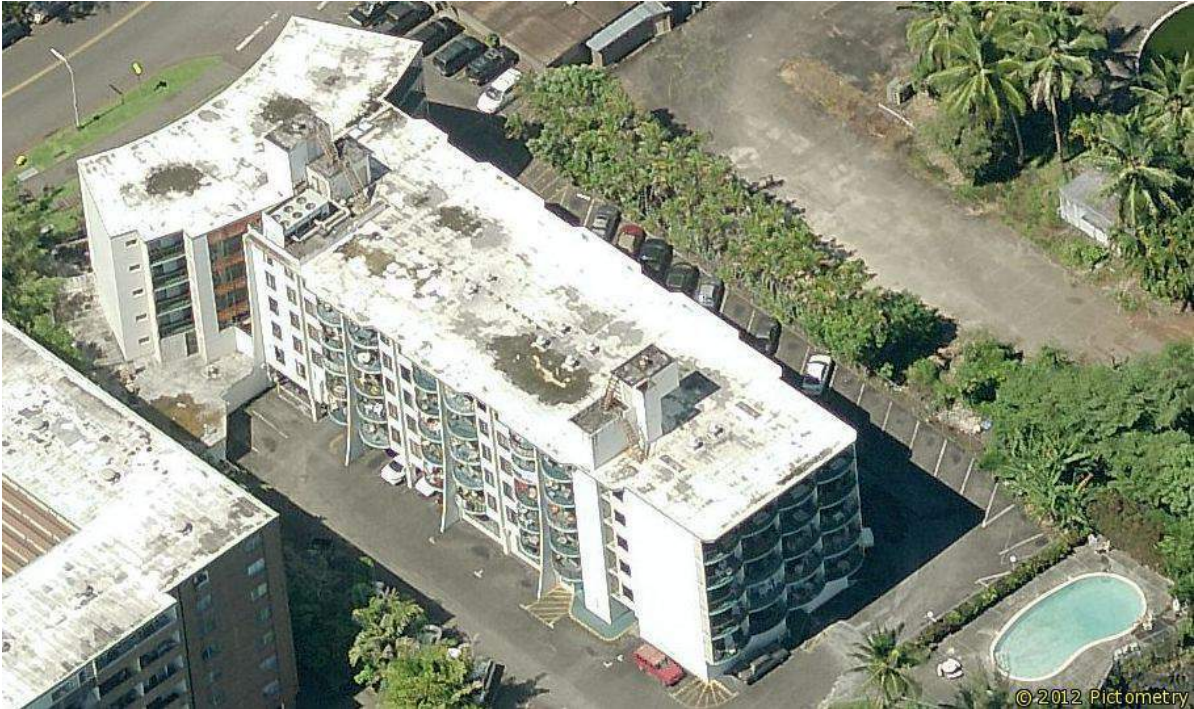
View from East
