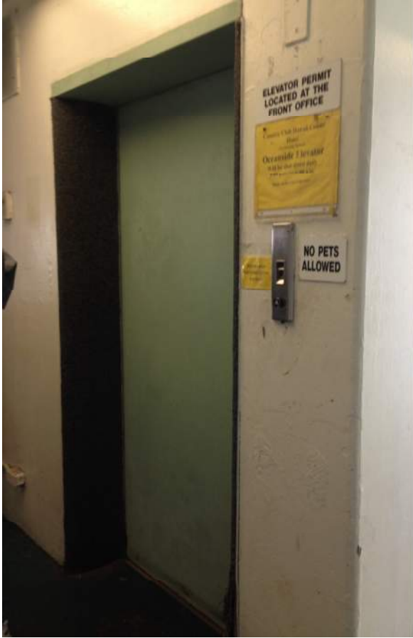
Photo 21: IMG_2461- Elevator in Lobby
