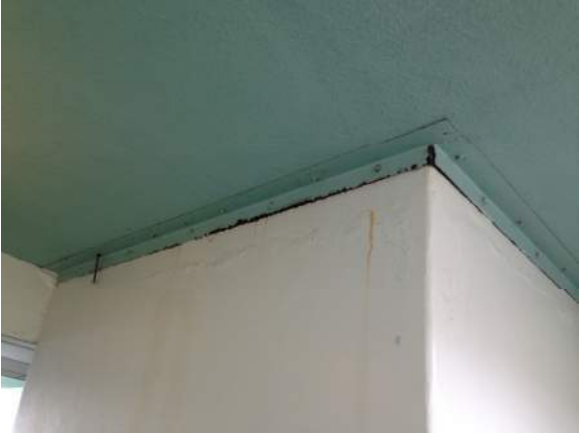
Photo 5: IMG_2507 – Rusting and loose bolt at slab ledger
