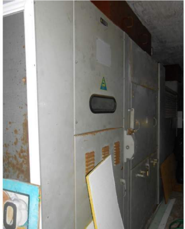
Photo 14: DSCN0451- Old electrical transformer, no longer in use
