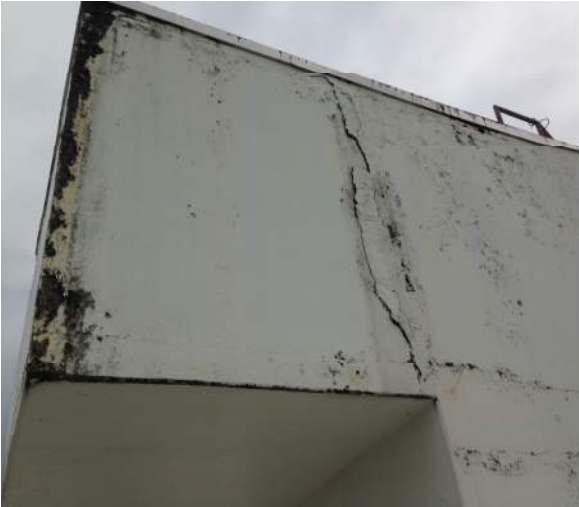
Photo 7: IMG_2491 – Spalling and cracking at Elevator Room
