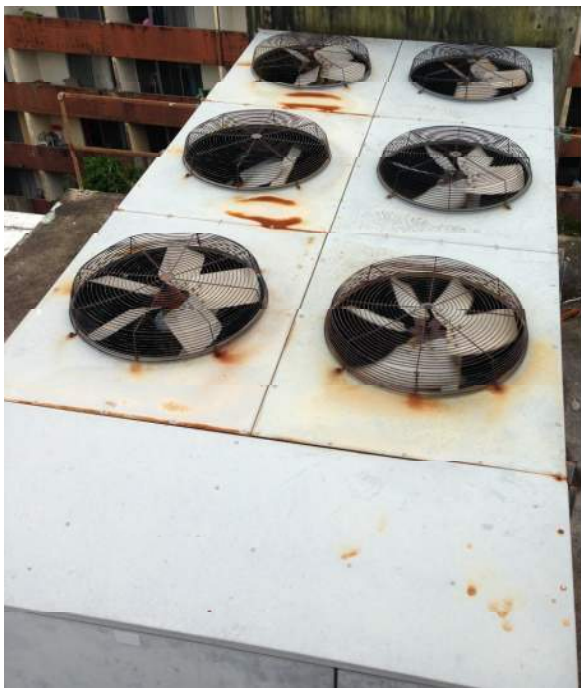
Photo 15: IMG_2489 – Air cooled chiller unit
