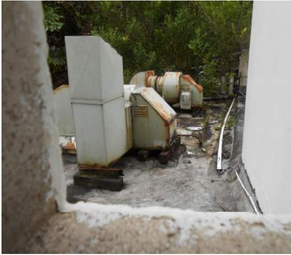
Photo 17: DSCN0479 – Defunct restaurant equipment
