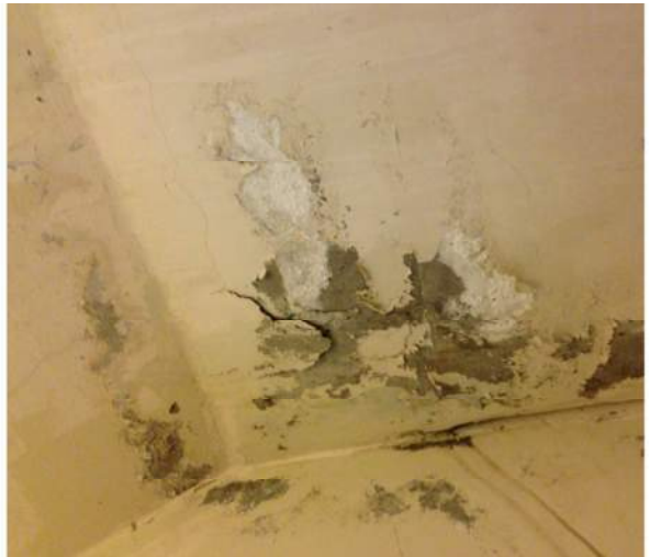
Photo 4: IMG_2494– Concrete slab spalling and efflorescence in stairwell
