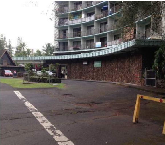
Photo 3: IMG_2447– Deteriorated pavement at drop off area
