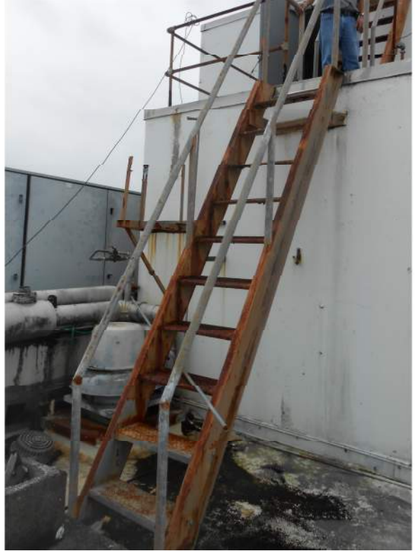
Photo 10: DSCN0471 – Roof stair rusting
